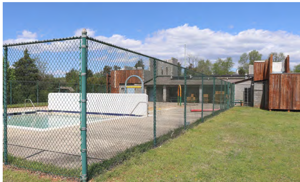
The castle facade to the Sharp pool entrance adds surprise and character to the landscape, but the pool and splash pad are inadequate for the Cub Adventure Camp needs.
