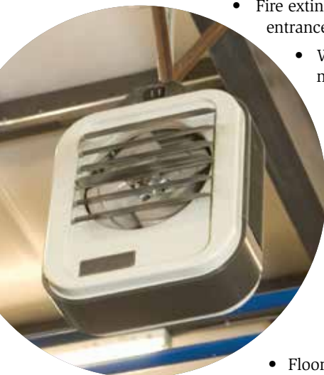
Ceiling-mounted heaters leave clear working space below.
